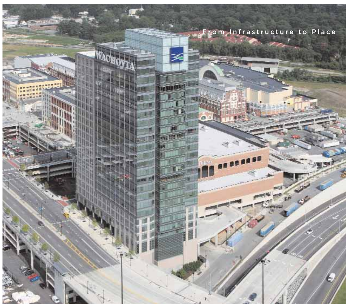
Parking vehicles underground offers an opportunity for a more positive use of land above ground. In Atlanta, Georgia’s Atlantic Station, a large structure was constructed to accommodate parking and utilities on the original ground level of the former Atlantic steelworks, and above it are the streets and buildings of the central hub of the new neighborhood.
